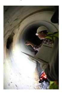
...and access cuts that allow workers (and excess storm flow) to travel between the larger 72-inch main pipes.
