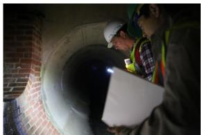
This is where storm water runoff collected from a number of streets along the Maple Avenue corridor to the south joins the main pipe we are traveling through. While the rest of the system is made of reinforced concrete pipe, most of these junctions are brick.
